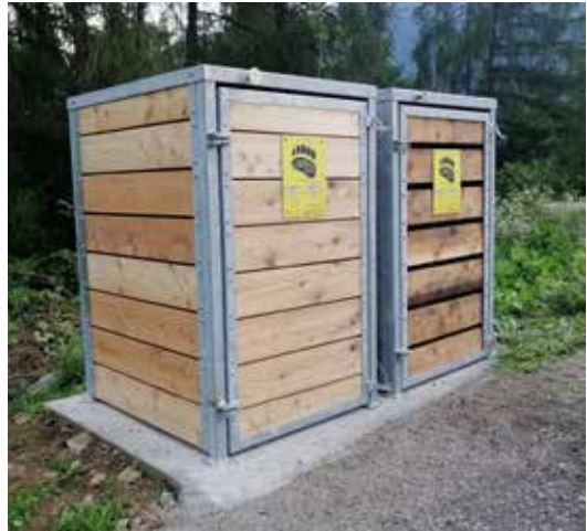
Photo 29 – The first two bear-proof structure prototypes initially positioned in Val di Sole to protect organic waste bins. (M. Benvenuti, APT Wildlife Department Archives)
