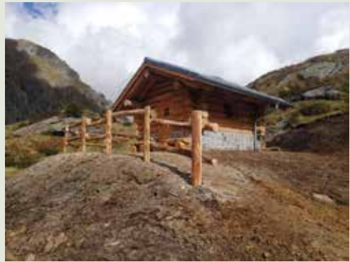
Figure C – Shelter built by Borgo Valsugana FDO at Sette Laghi, Torcegno. (R. Dalledonne, APT Forestry Department Archives)
